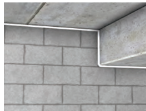
Construction joints
